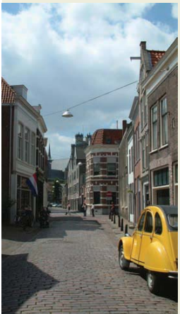
Varkenmarkt 46a, architect Th. Van Halwij
